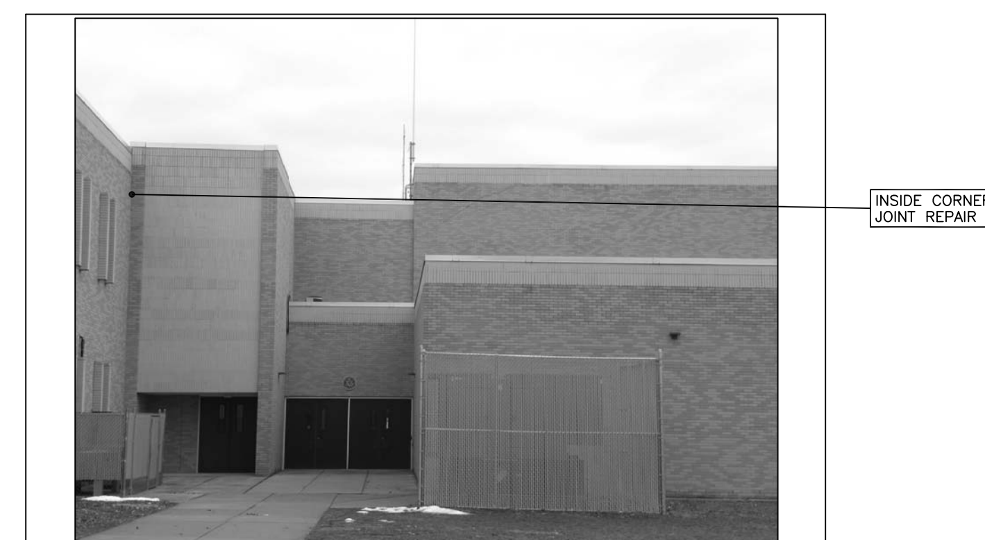
REPAIR @ INSIDE CORNER VERTICAL JOINT DETAIL
